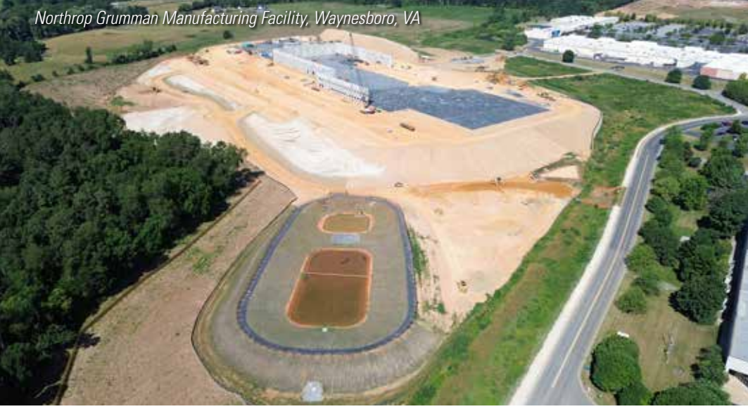
Northrop Grumman Manufacturing Facility, Waynesboro, VA
