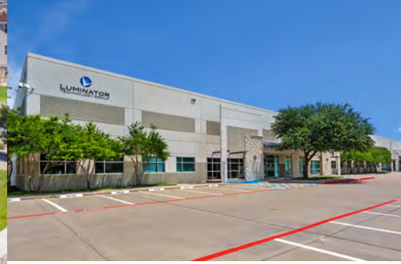
Project Colt - 2280-2300 NW 30 th Place, Pompano Beach, FL
