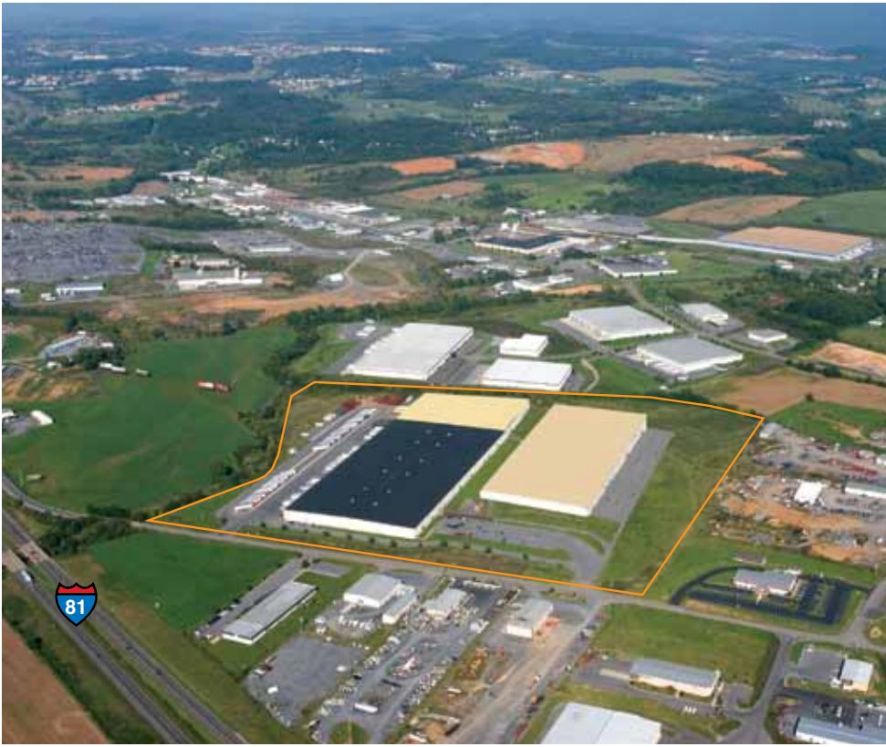
I-81 Distribution Center, Harrisonburg, VA
